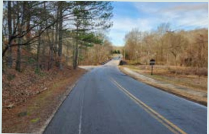
Looking West on Klondike Road, roadway stormwater runoff is collected in south side ditch, but then sheet flows at the entrance of Everett Park
