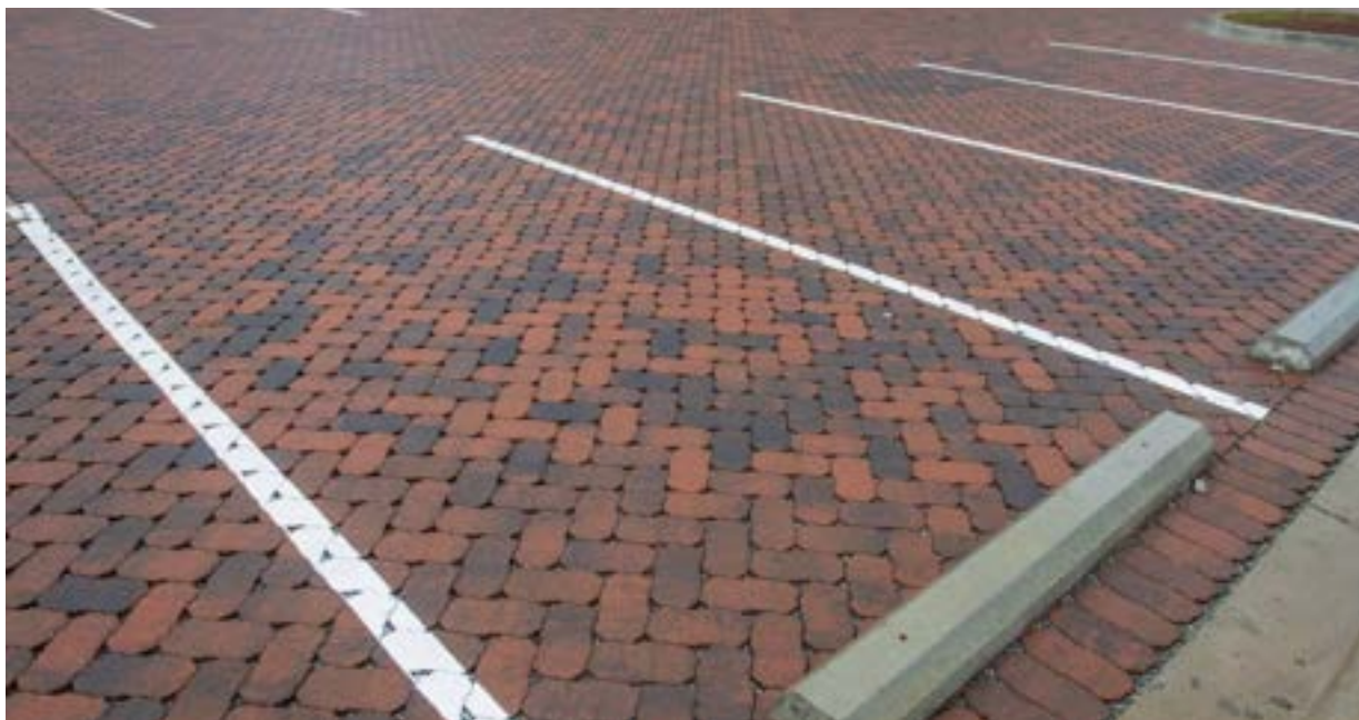
Proposed Permeable Pavement for Parking Area
